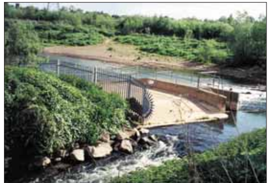
Fish pass at Powick Weir
